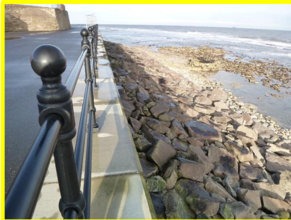
Shallow profile rock armour but shows good interlock (/C0303C02)
