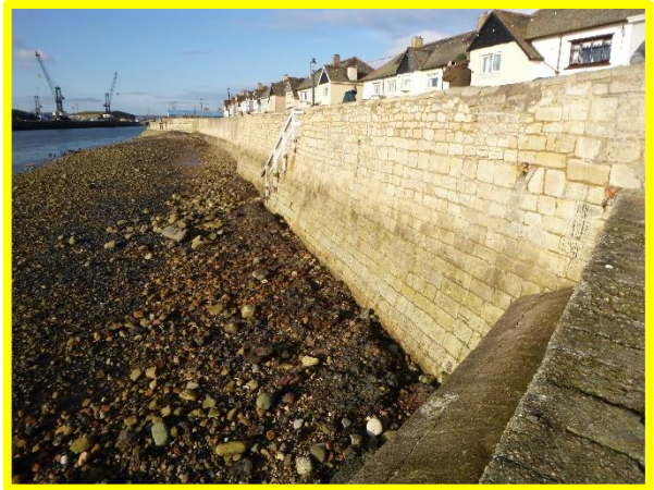
Wall generally in fair condition (/C0401C35)
