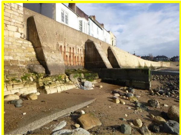
Recently constructed outfall and abutment. (/C0401C35)
