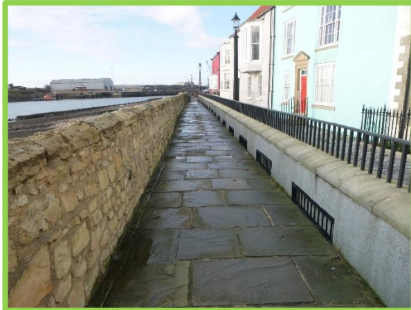
Repaired footpath and flood wall in good condition (/C0401C35)
