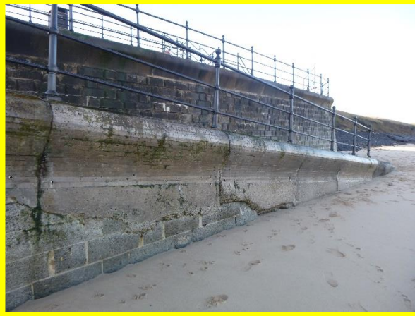
Historic repair to access ramp coping stone in fair condition (/C0303C01)
