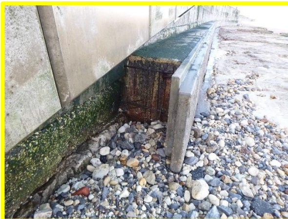
Outflanked toe feature (/C0303C01)
