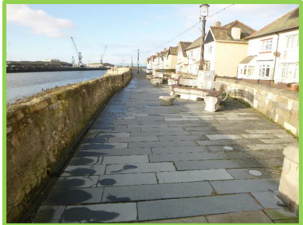
Promenade and rear wall in good condition (/C0401C35)
