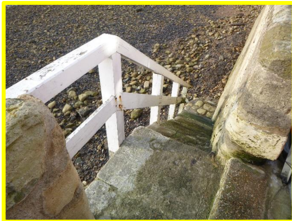
Beach access steps (/C0401C35)
