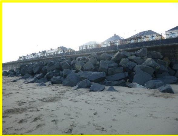
Rock armour in fair condition (/C0303C01)
