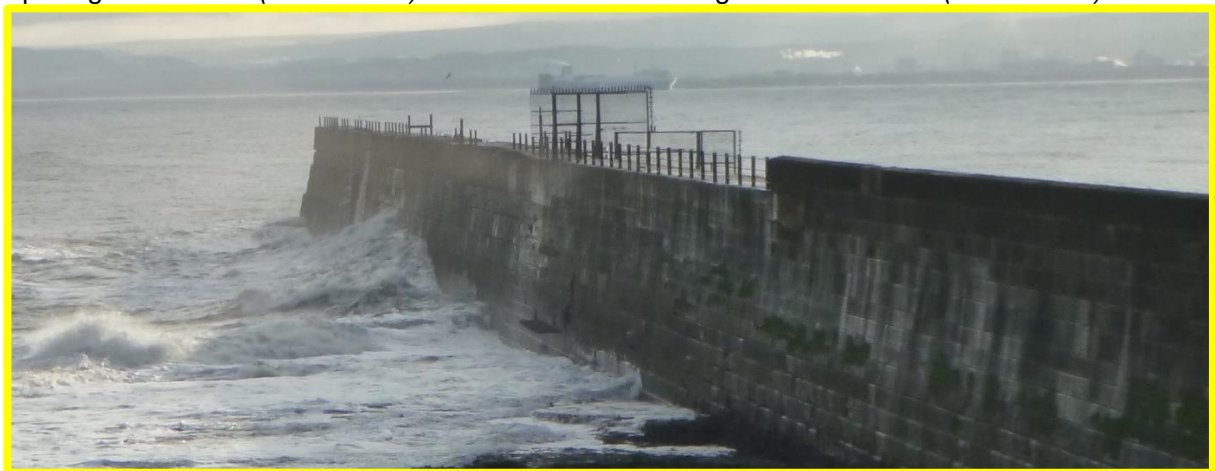
Northern aspect of the Heugh Breakwater (/C0401C01)
